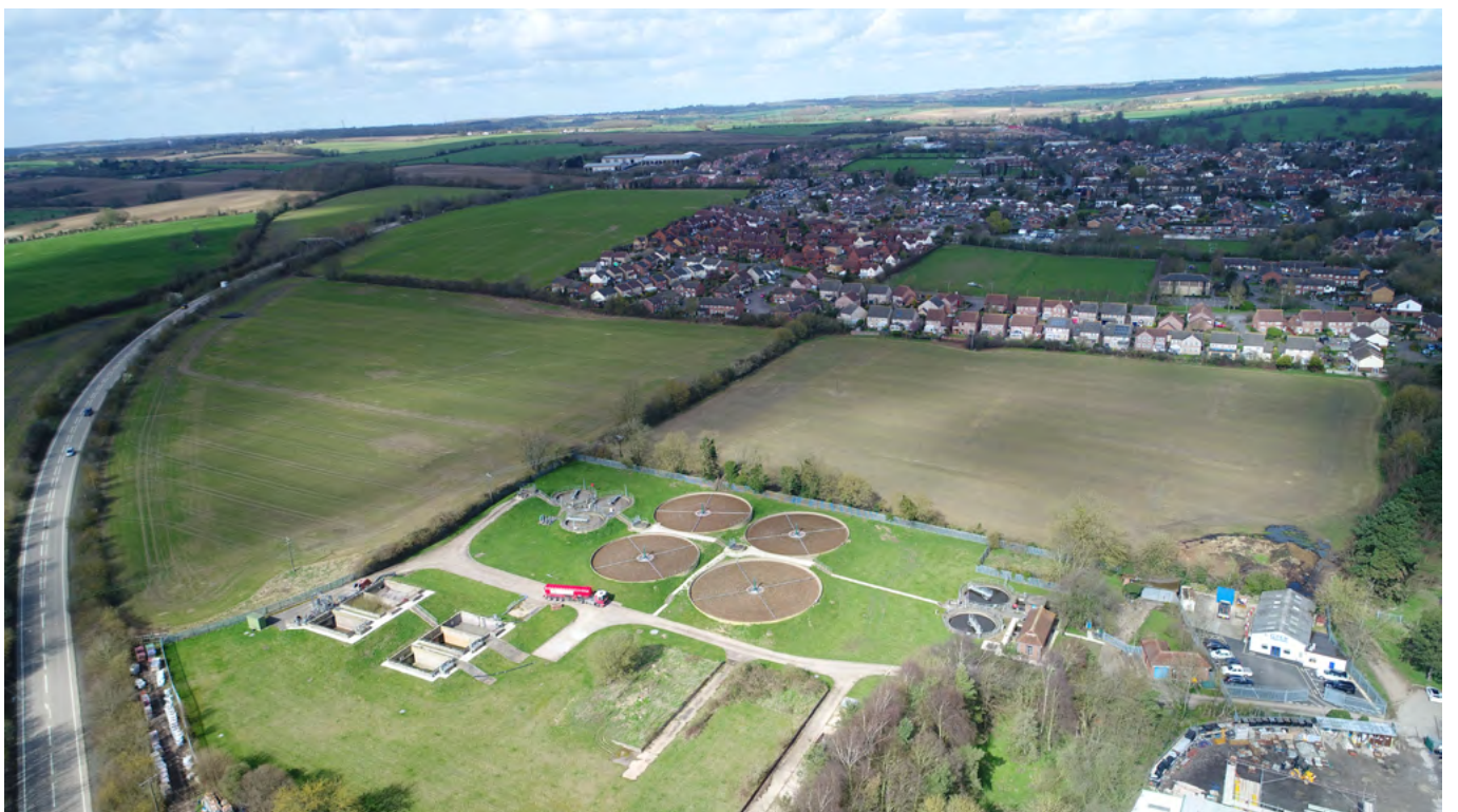
Aerial View Looking North West (March 2017)
