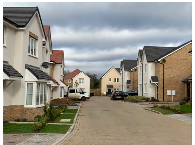
Shared surfaces to streets and minimal use of tarmacadam. A mix of render, buff brick and weatherboard.
